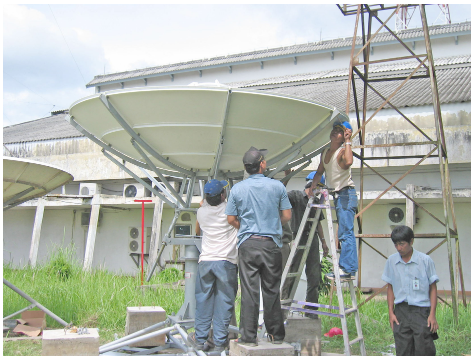
Installation of the network antenna at the Palembang radio station in rural Indonesia.
