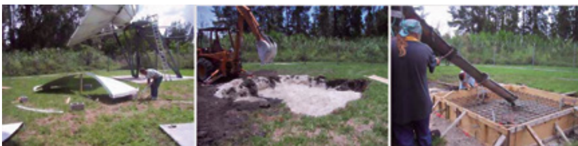
Installing a VSAT System, from left to right: Installer starts the assembly of an Andrew 4.5m antenna—the foundation for the base is excavated—the concrete for the base is poured. Photos courtesy of New Era Systems.
