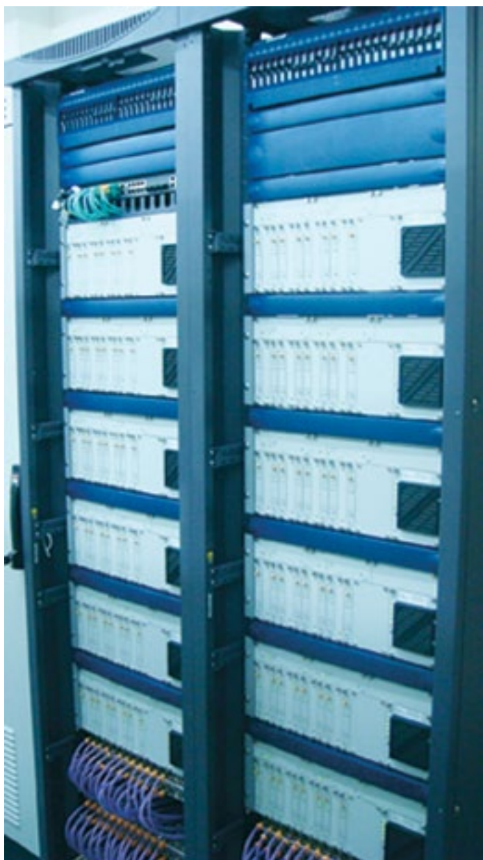
DEV2190 L-Band Distribution systems in IPTV super head end downlink at Etisalat, UAE
