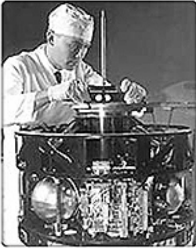
Engineer Dave Kamm aligns Syncom before its orbital alignment: synchronous with Earth's rotation at 22,300 miles altitude.
